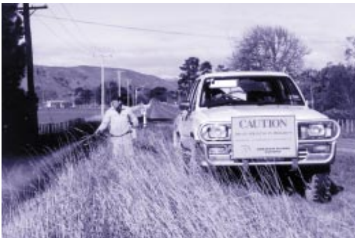
Drain maintenance by herbicide spraying
