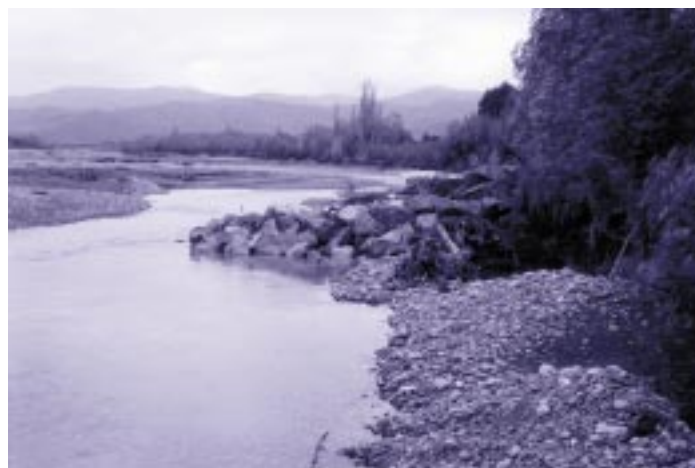
Rock groynes – Waiohine River
