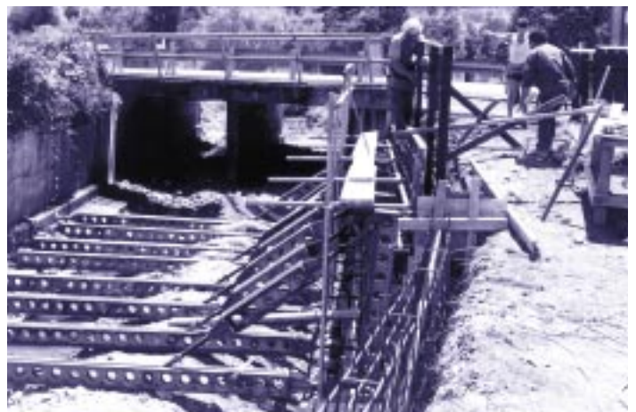
Retaining wall construction – Donald's Creek, Featherston
