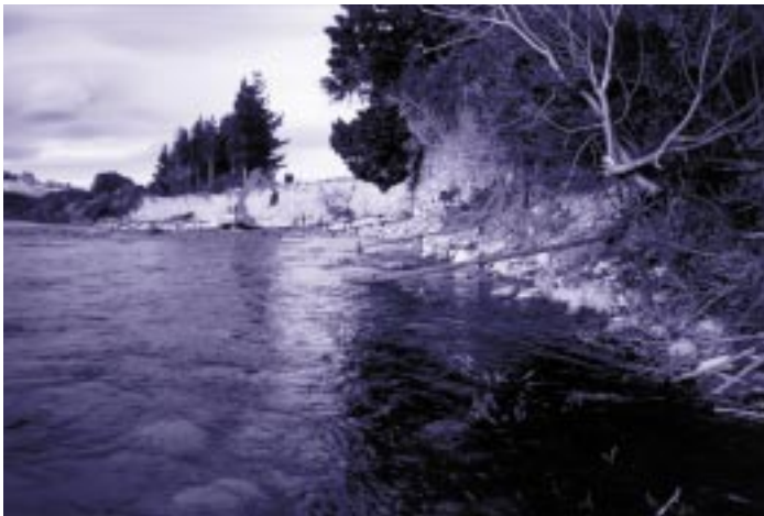
Rail groyne construction – Waingawa River
