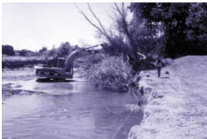
Willow cabling – Waipoua River
