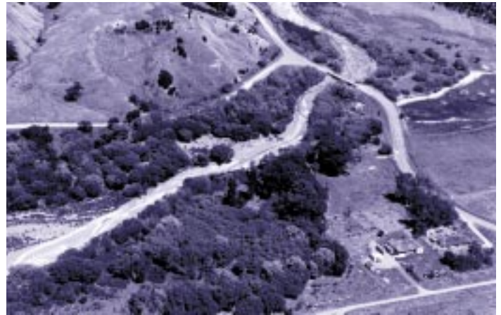
Stoney Creek Bridge at Tukurumuri
