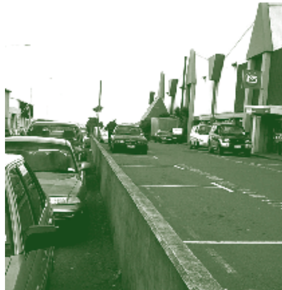
An example of a voluntary action by NZ Post in Petone. You can see by the carpark on the right hand side of the photo that the site has been raised by over 1 metre.
