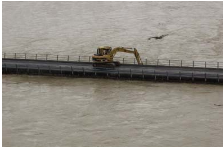
Cleaning debris from the Waihenga Bridge. February 2004 flood.
