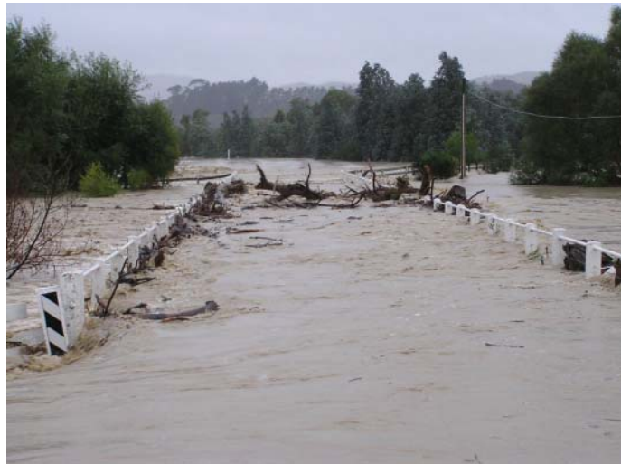
The Ponatahi Bridge on 16 February 2004.
