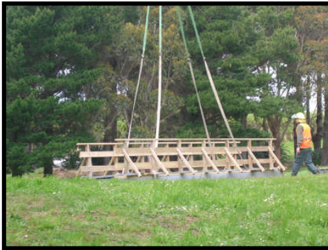
The bridge is stropped up...
