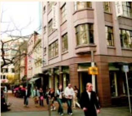
Mixed use – A mix of retail outlets, cafes, bars and professional offices attracts people to Vulcan Lane in Auckland at all times of the day and night.
