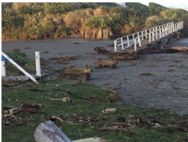
Paekakariki footbridge damaged by sea action and debris.
