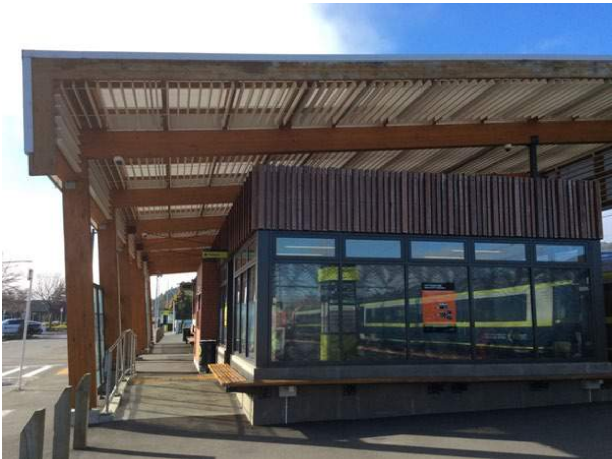
Figure 36: Upper Hutt Station Building – rebuilt in 2015.
