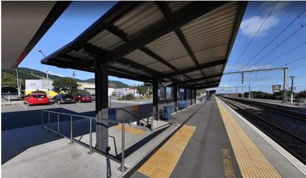
Figure 38: Shelter at Paraparaumu
