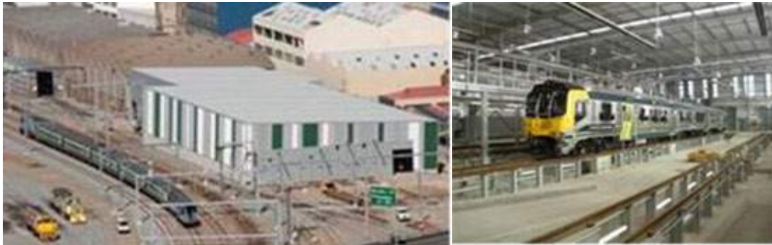
Figure 68: EMU maintenance depot facility
