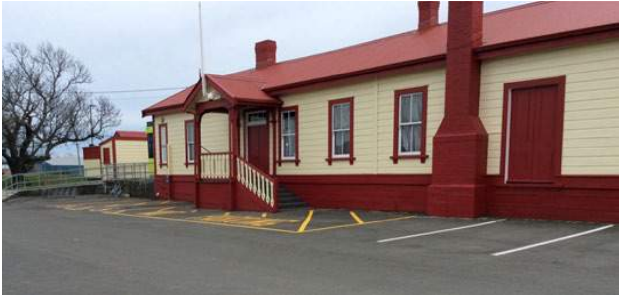
Figure 37: Carterton Station Building
