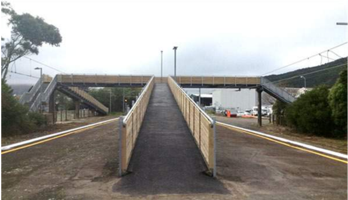
Figure 61: Wingate North pedestrian overbridge – post seismic strengthening improvements
