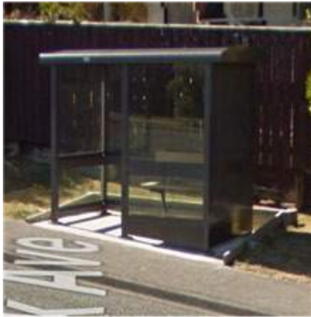
Figure 71: CAM bus shelter
