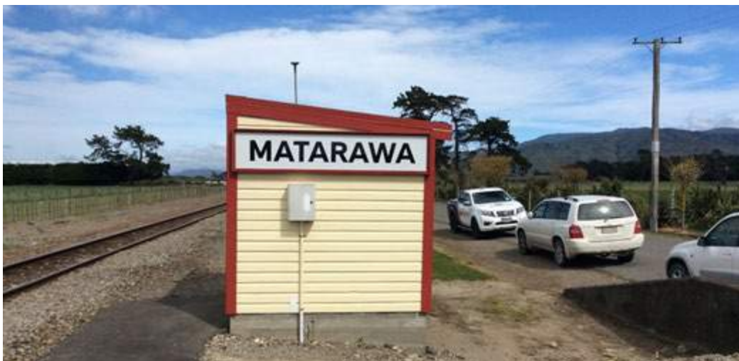
Figure 39: Shelter at Matarawa
