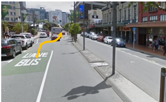
Figure 18: Weaving on the Northbound Approach to Taranaki Street
