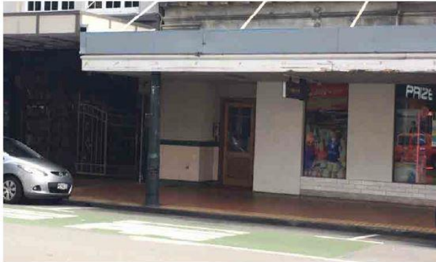
Figure 29: Example of Unattractive Built Edge near Te Aro Park
