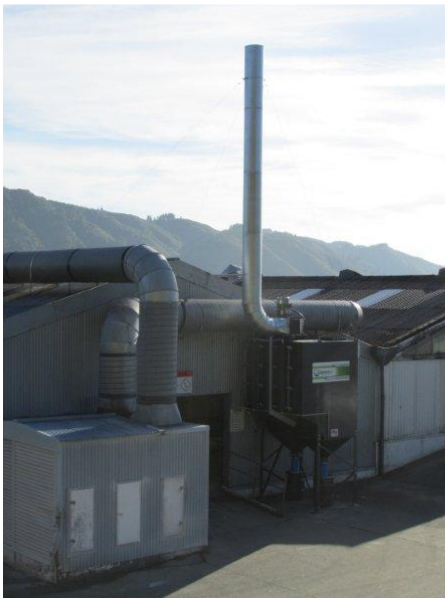
Figure 3-1: Cartridge filter and discharge stack
