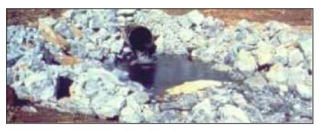
Fig 2.3.1: Typical Coastal Outfall Under Construction.
