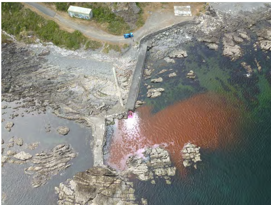
Figure A.3 Drone image of the dye test at 10:32 on the 29 th November 2017.
