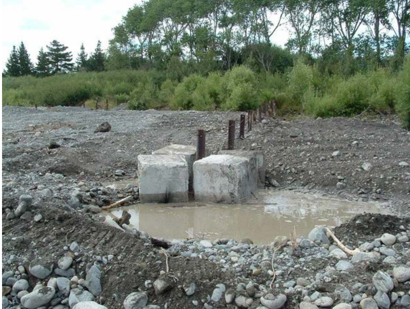
Figure 5-3: Completed debris fence, Otaki River.
