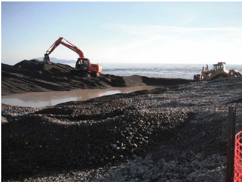
Figure 5-7: Diversion cut, Otaki River Mouth
