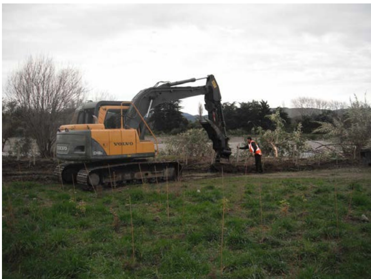
Figure 5-4: Willow pole planting (note native plantings in foreground)
