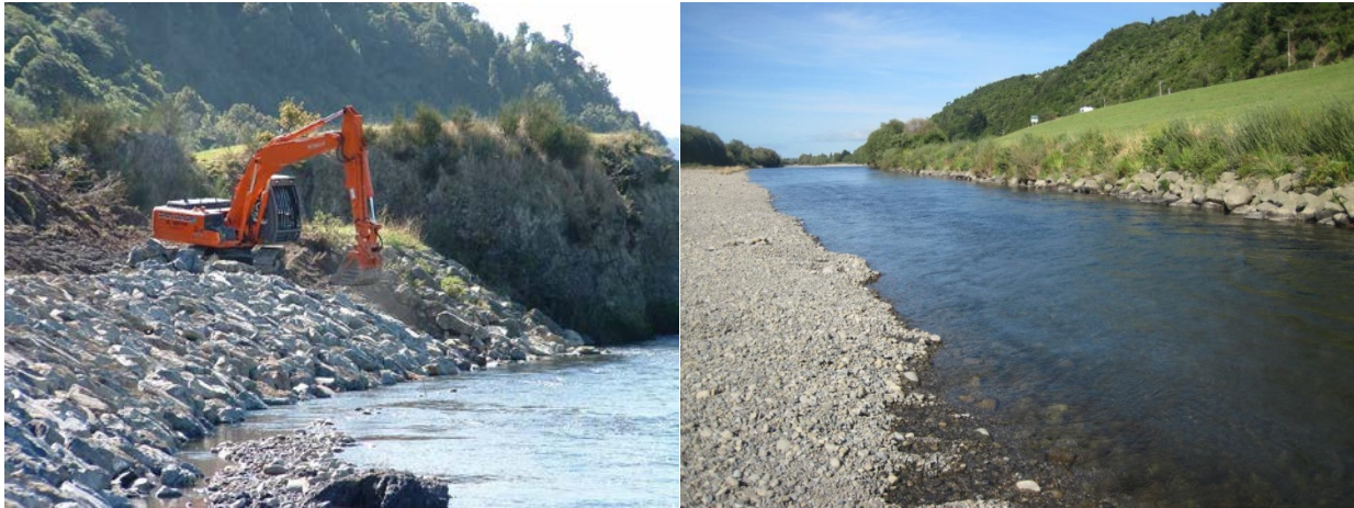
Figure 5-2: Rock rip-rap linings, Hutt River
