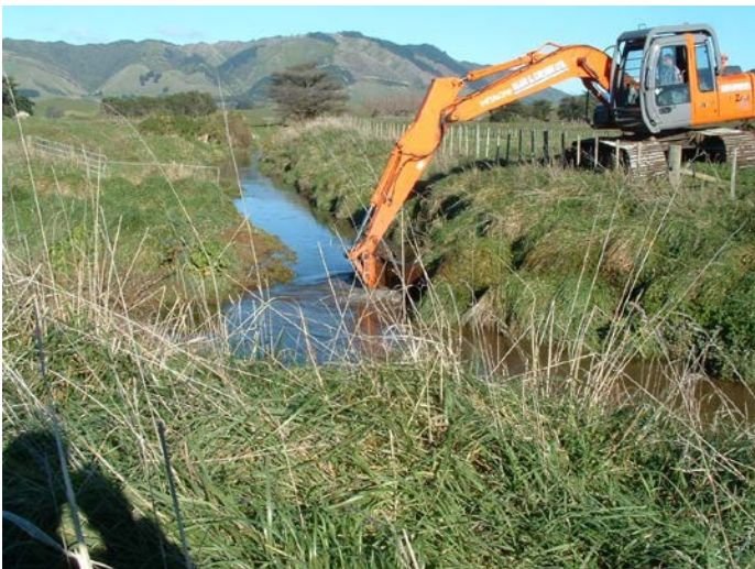
Figure 5-5: Vegetation and silt clearing on the Pahiko Drain
