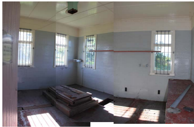
Engine room. This had the power boards and was also where the light was turned on and off every day. The Lister powered alternator was in there also and was a back-up to the mains power.
