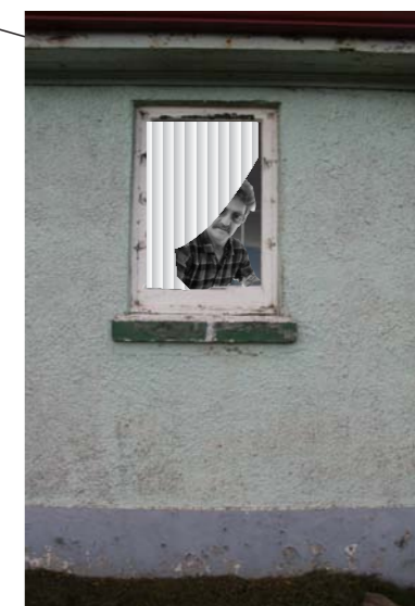
store-room, with cupboards lining the wall on the left hand side as you go in. There was most things required for the station maintenance stored in there. Paint, methylated spirits, tap washers, nails, screws, hinges, light bulbs, fence wire etc.
