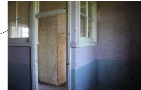
Fuel store. The lawnmower and other larger implements were also stored there. The fuel was petrol for the mower and diesel for the Lister engines (The generator and also the water pump at the Wainui River).
