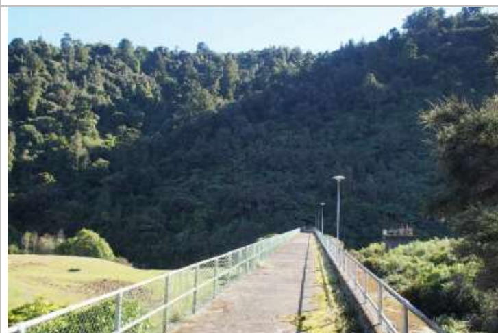
Photo 4: Western Spur from dam wall.
