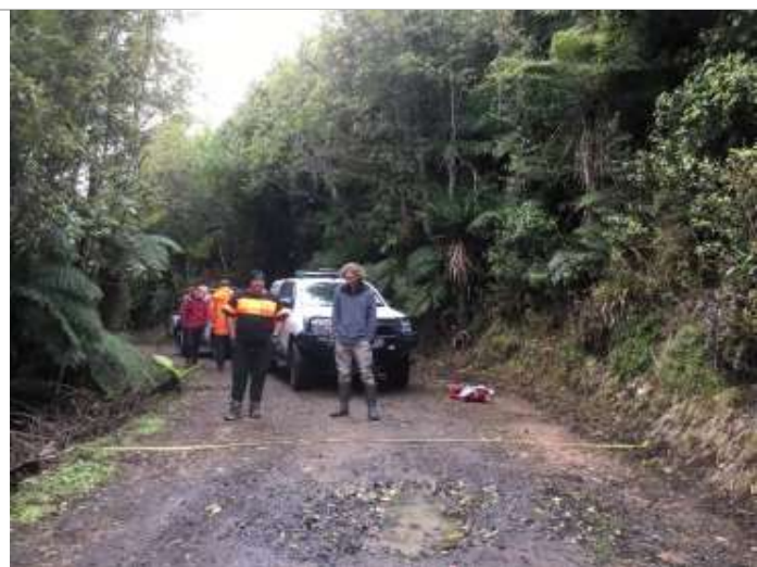
Photo 16: Existing access track at eastern ridgeline. Formed width is 5.9m. Lengths of this track will require widening to provide for both large vehicles and the fence.
