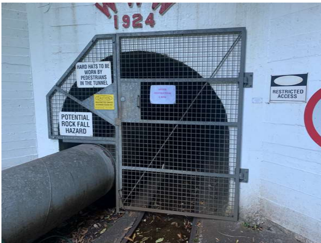
Figure 15. Orongorongo tunnel. Photo Ricky Clarkson
