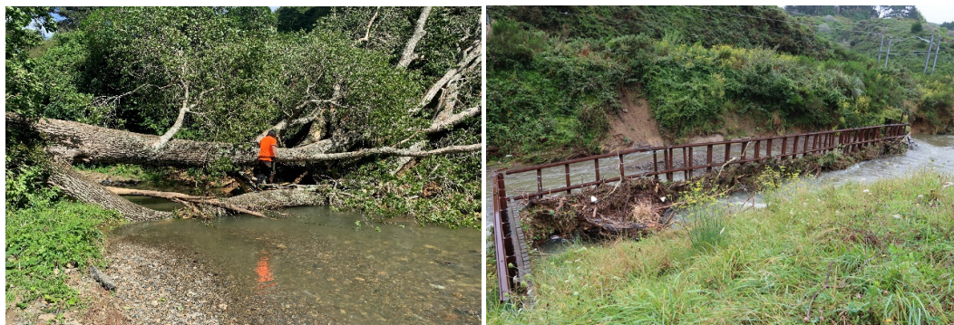
Photos of fallen trees on the Porirua Stream (left) and the damaged debris arrestor (right).
