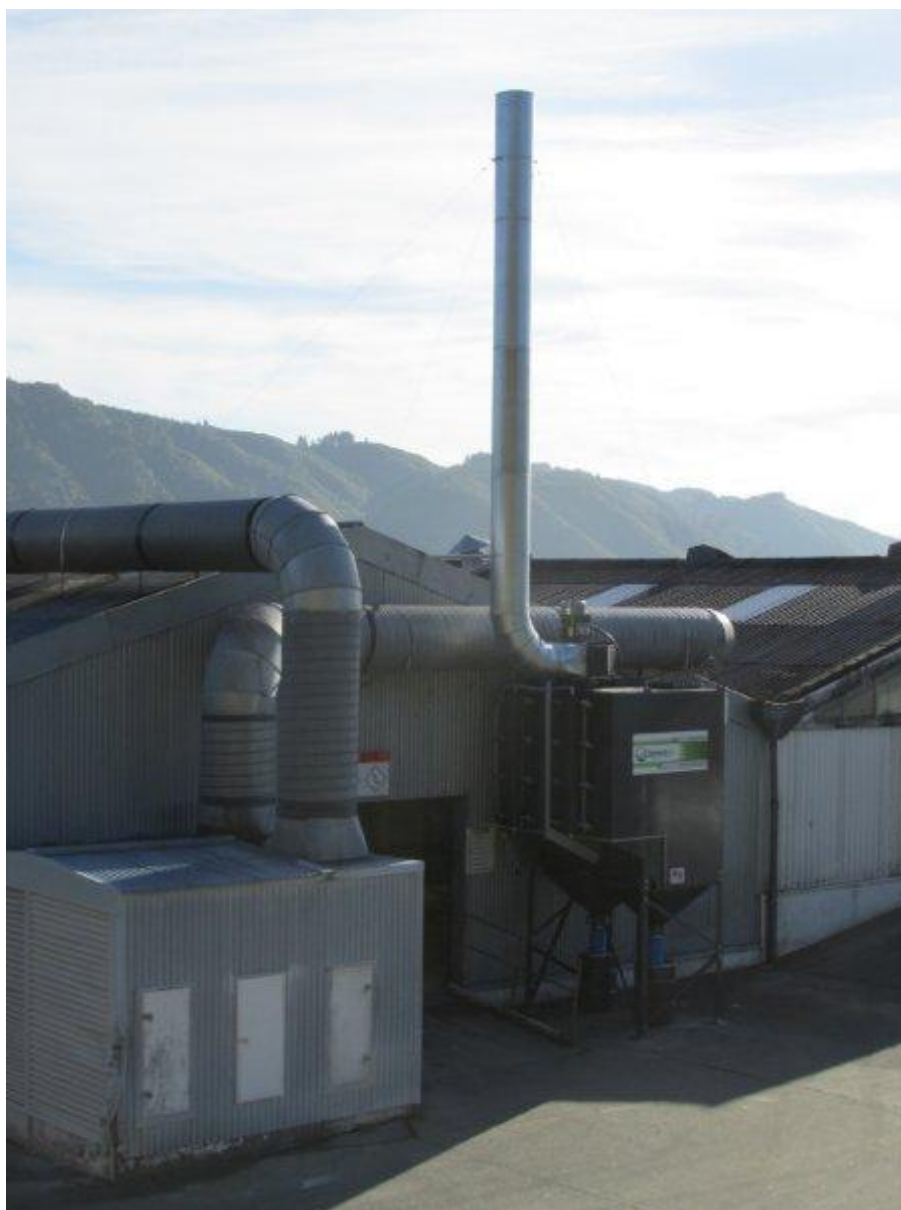
Figure 3-1: Cartridge filter and discharge stack
