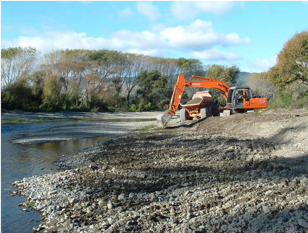
Figure 6: 'Dry' gravel extraction (example from Waikanae River)
