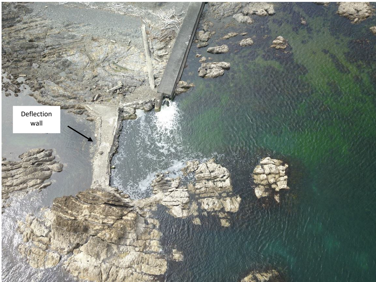
Figure 2-3: Aerial view of the wastewater outfall at Rukutane Point (from Cawthron 2018)
