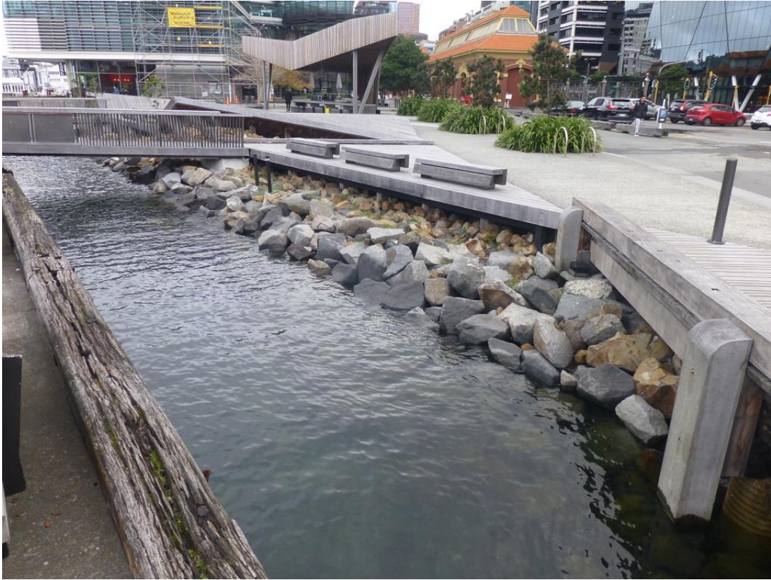
Northern end of the rip-rap, edge of the Tug Wharf on the left, Kumutoto Park north in the distance.
