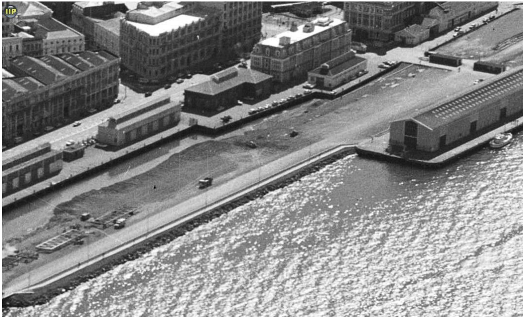
Above: Two details of an image taken in 1971 showing the formation of the new harbour edge, including the walkway from Tug Wharf (top). (EP-1971-5004-F 1971-1, Alexander Turnbull Library)
