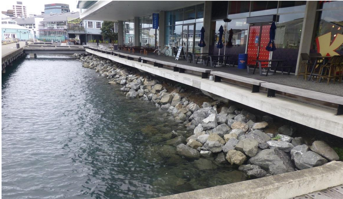
3 The central section of the rip-rap, running alongside the Meridian Building.
