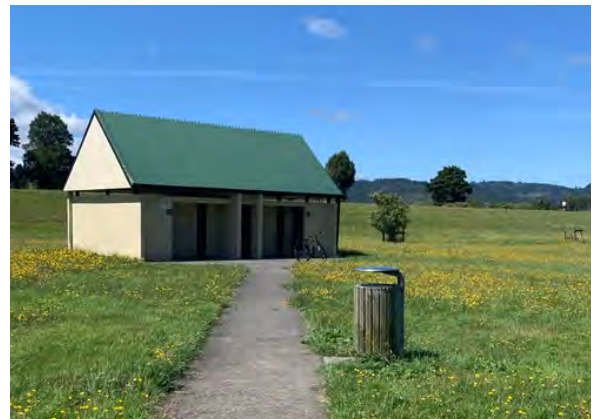
Figure 45. Bathroom at Moonshine Bridge Park
