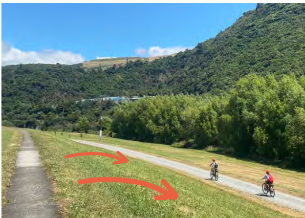
Figure 17. Photo taken on top of a stop bank with arrows depicting how the slope directs water back into the Corridor during a flooding event.
