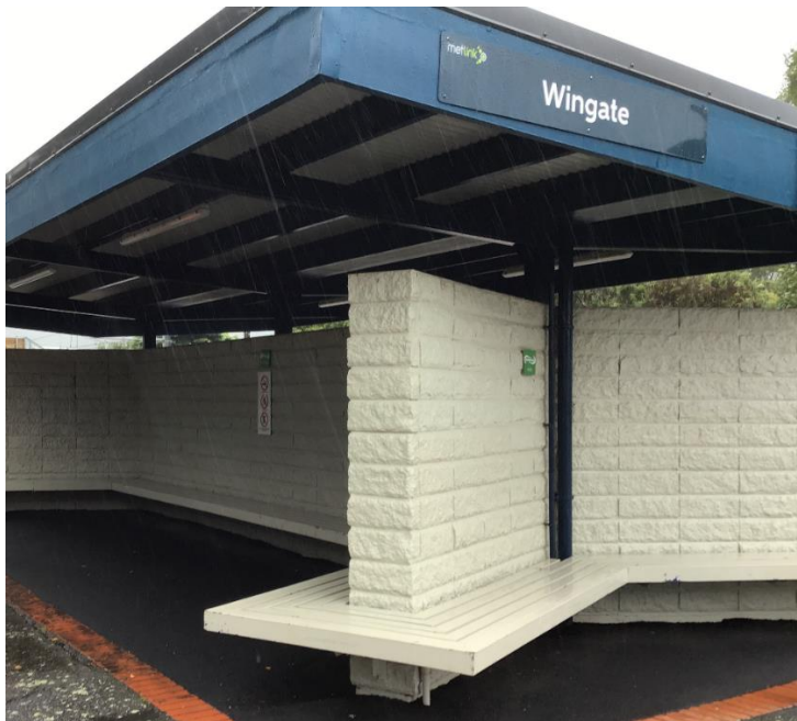
Figure 35: Previous Wingate shelter
