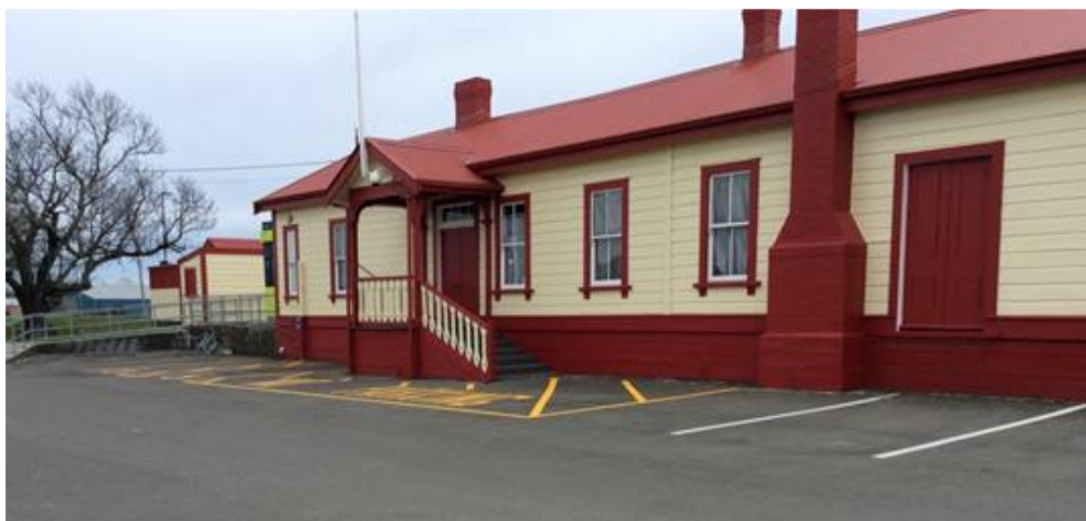
Figure 34: Carterton Station building
