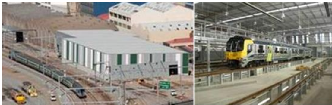
Figure 67: EMU maintenance depot facility
