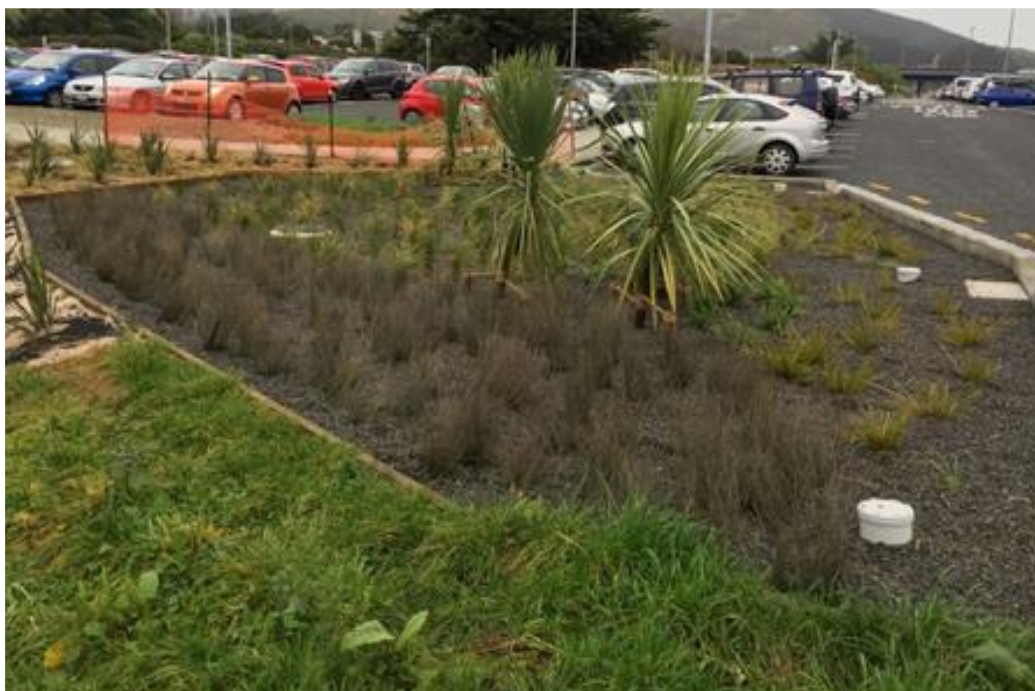
Figure 42: Porirua Station Park and Ride northern rain garden
